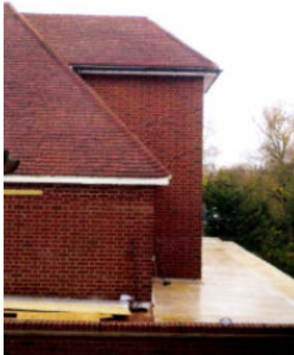
Part of side elevation seen from No 20
